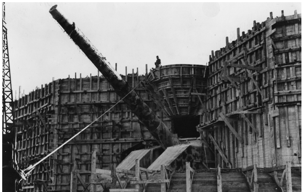
Construction of a gun emplacement at the Atlantic Wall. The defensive installations reached from Norway to the border of Spain and were supposed to make any attack from the sea impossible. (34.11)
